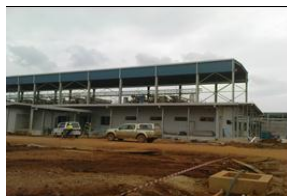
C2 – Operation Control Room
