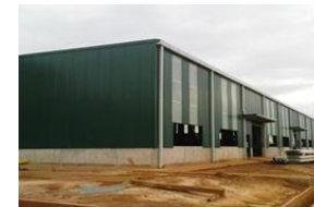
C6 – Production Storage
